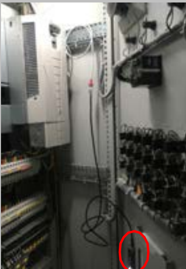
Thermal camera installation position
